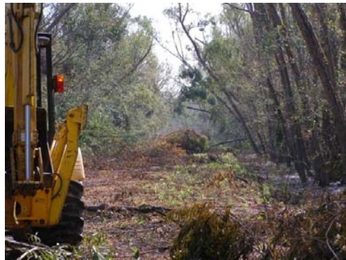
BC Brine Disposal Road
