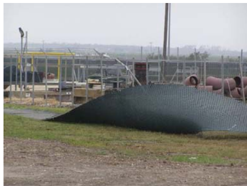
BM Fence Around Laydown Yard
