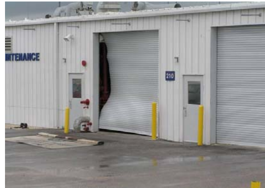
BM Maintenance Building
