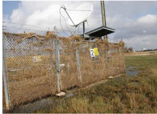
WH Meter Station Fence
