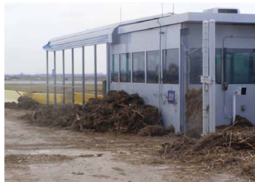
BH Debris Around Entry Portal
