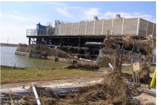
BH Raw Water Intake Structure
