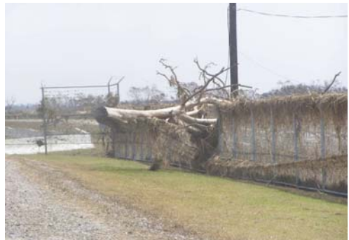
BH Fence Damage
