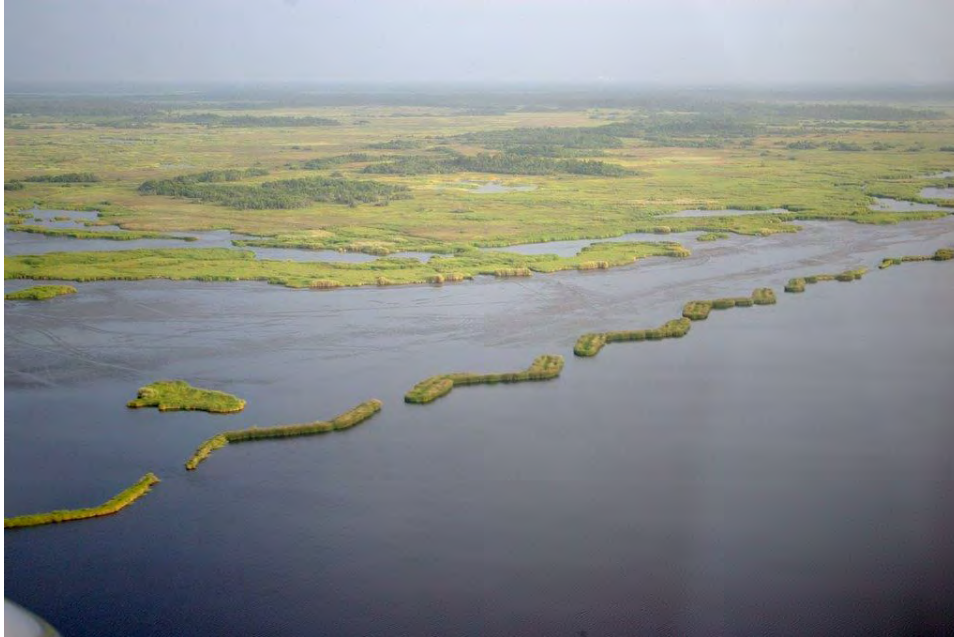
Exhibit 2 – Typical Terracing Project Constructed to Reduce Wave Fetch and Protect Existing Land. Source: Panoramio – Photos by stefkuna.
