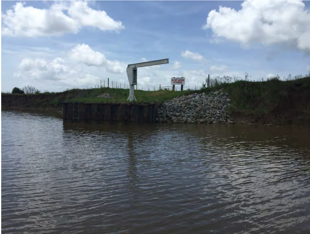
Photo 1 – WH-2 landing site showing bulkhead, ladder, and davit crane.
