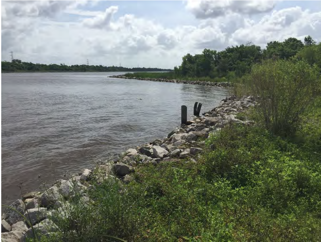
Photo 3 – WH-5 landing site with rip-rap stabilized bank.
