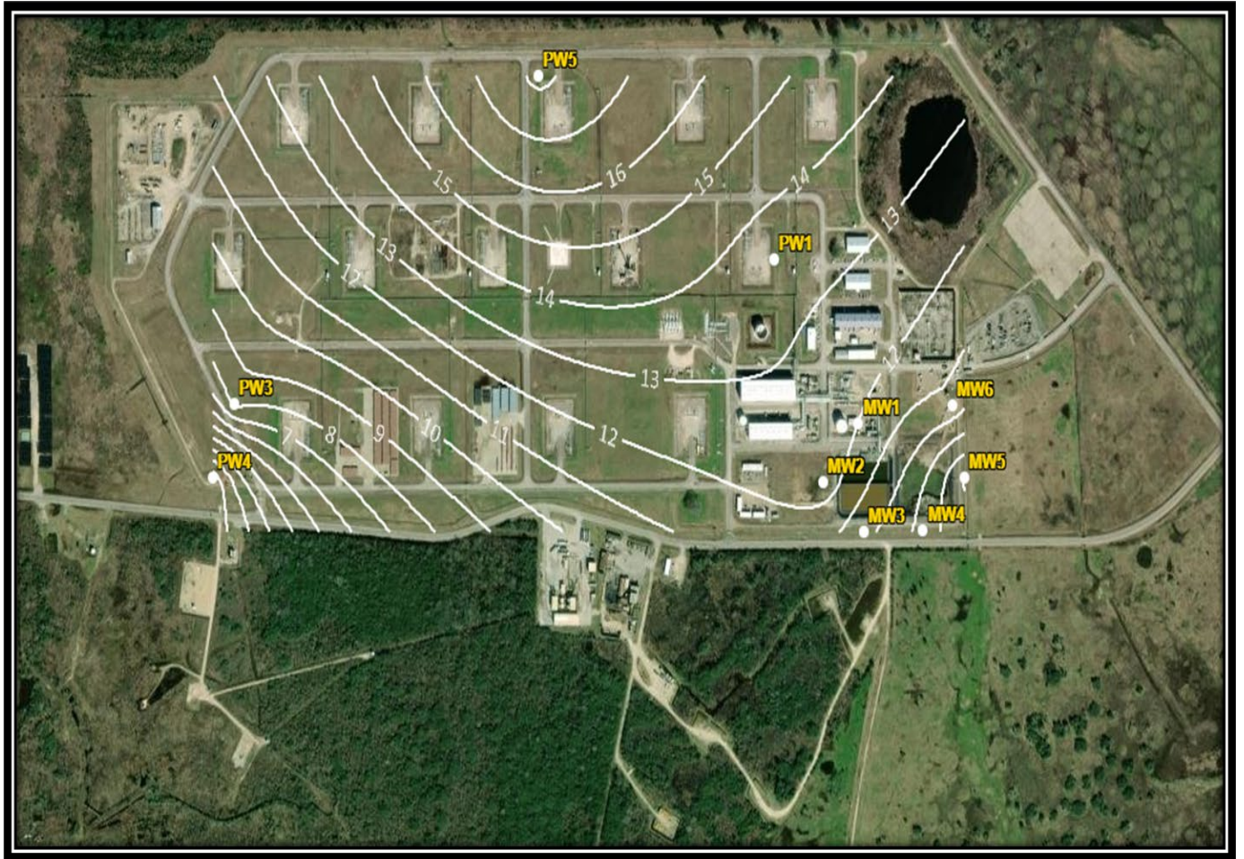
Figure C-5. Big Hill Ground Water Contoured Elevations June 2023
