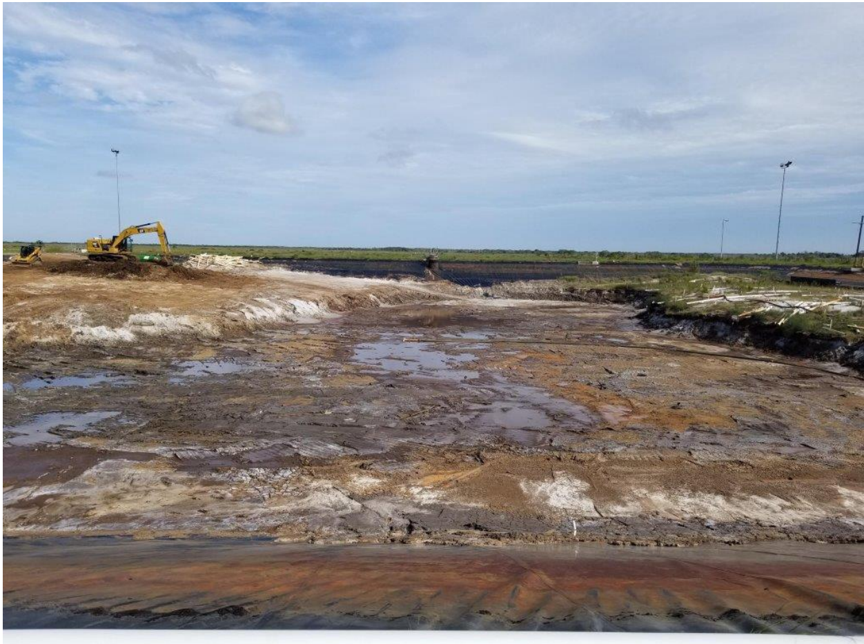
Figure 2-3 BH Brine Pond 9 Post Sediment Removal (10/24/2019)
