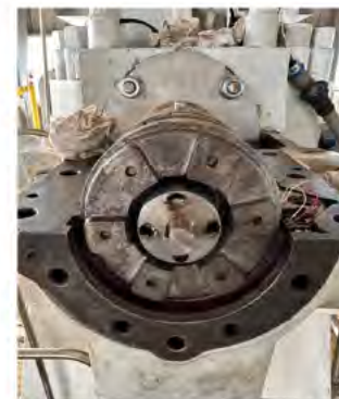
Replacement of Mechanical Seal for Brine Injection Pump BCP-213 by Site Maintenance
