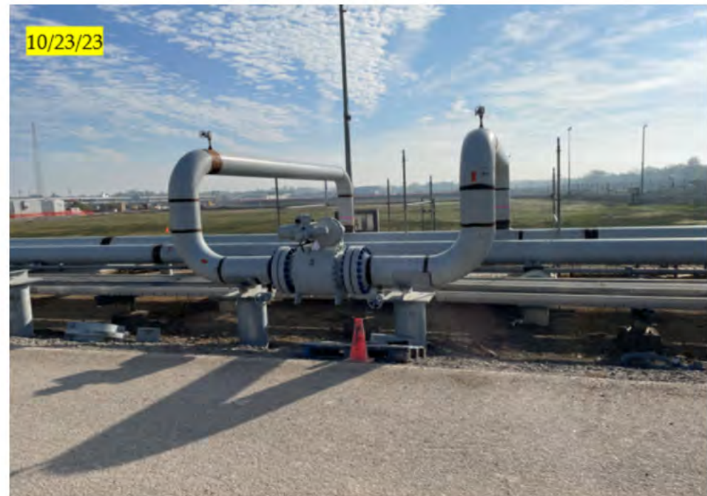
Pipe and valve installation at N/S Piperack
