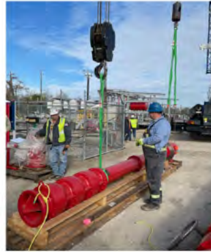
BC-LE-1759, New Fire Water Pump Installation at the Raw Water Intake Structure
