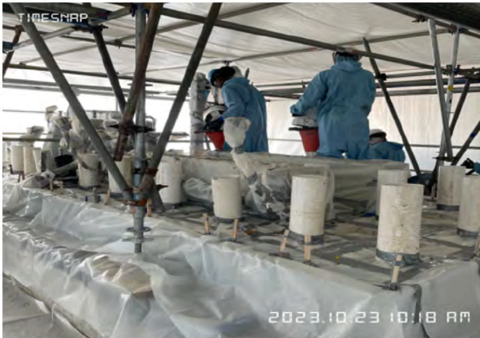
Grout installation at BCP-603 at HPPP
