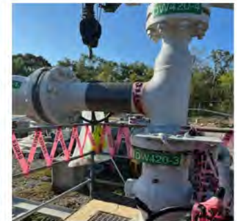
Brine Disposal Well #4's Tee Section removal by Site Maintenance
