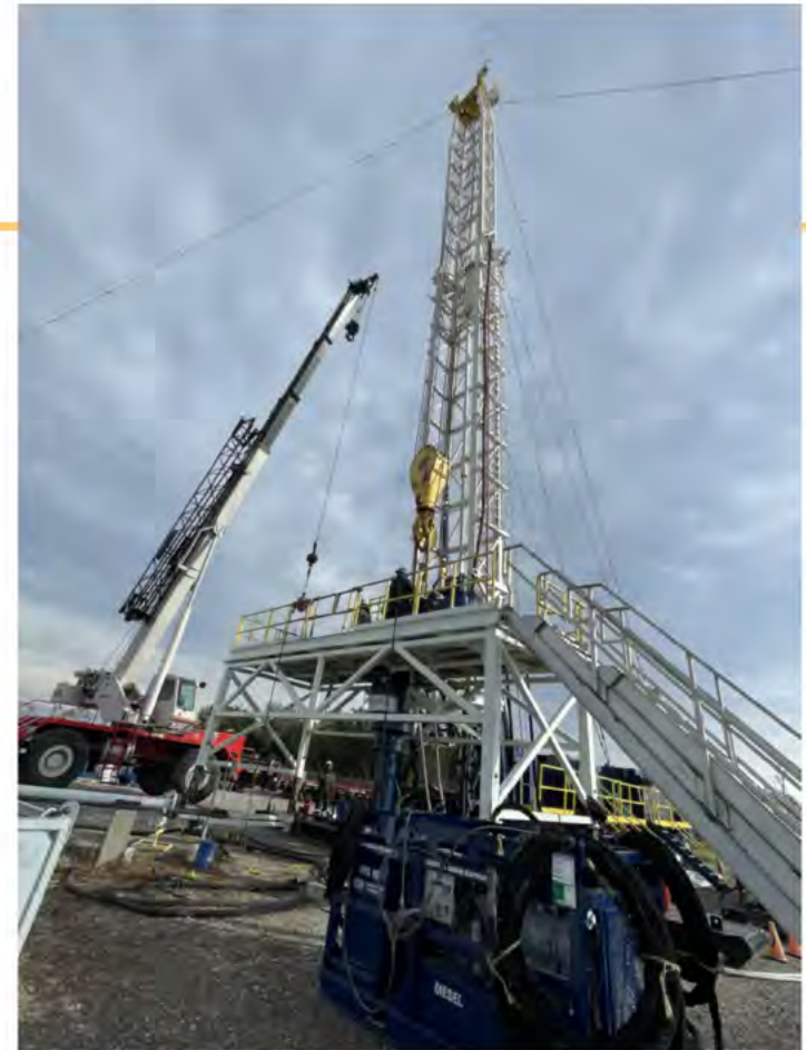
Workover Rig on BDW 1-A
