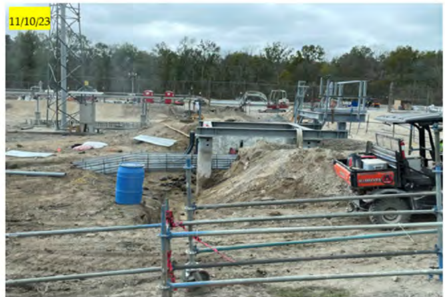
Installing of ductbank and steel at BDW#2
