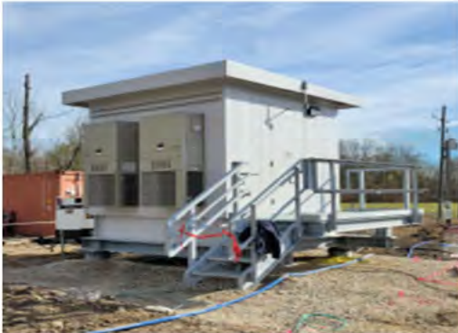
BC-LE-1759, FIB Building Installed at Disposal Well Pad #1
