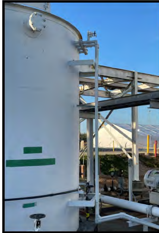
Seal Flush Pump Recirculation Line Replacement
