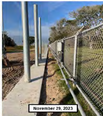
November 29, 2023 BH-LE-1735 – Completed fence posts and apron along North perimeter CWA-80
