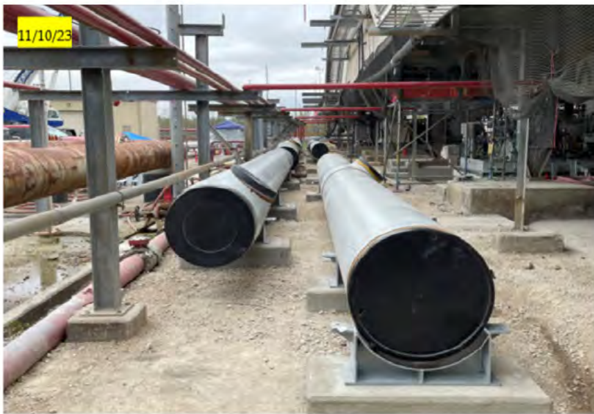
Reinstalled pipe headers for Raw Water Injection Pump (3)
