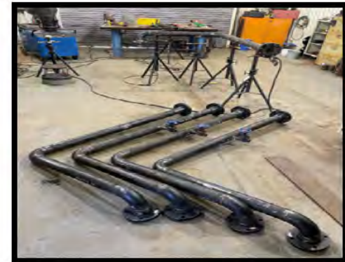
Traveling Screen Lines Fabricated on-site
