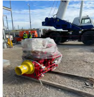
BC-LE-1759, New Fire Water Pump Installation at the Raw Water Intake Structure
