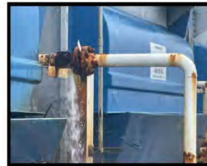
Leak at the Raw Water Intake Structure
