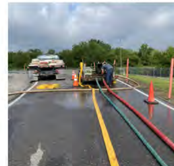
Annual Fire Hose testing
