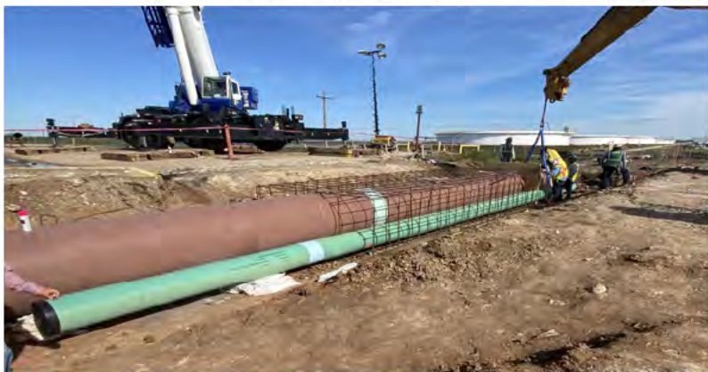
Piping and Duct Bank Placement
