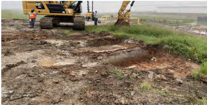
Excavating Old RW Line
