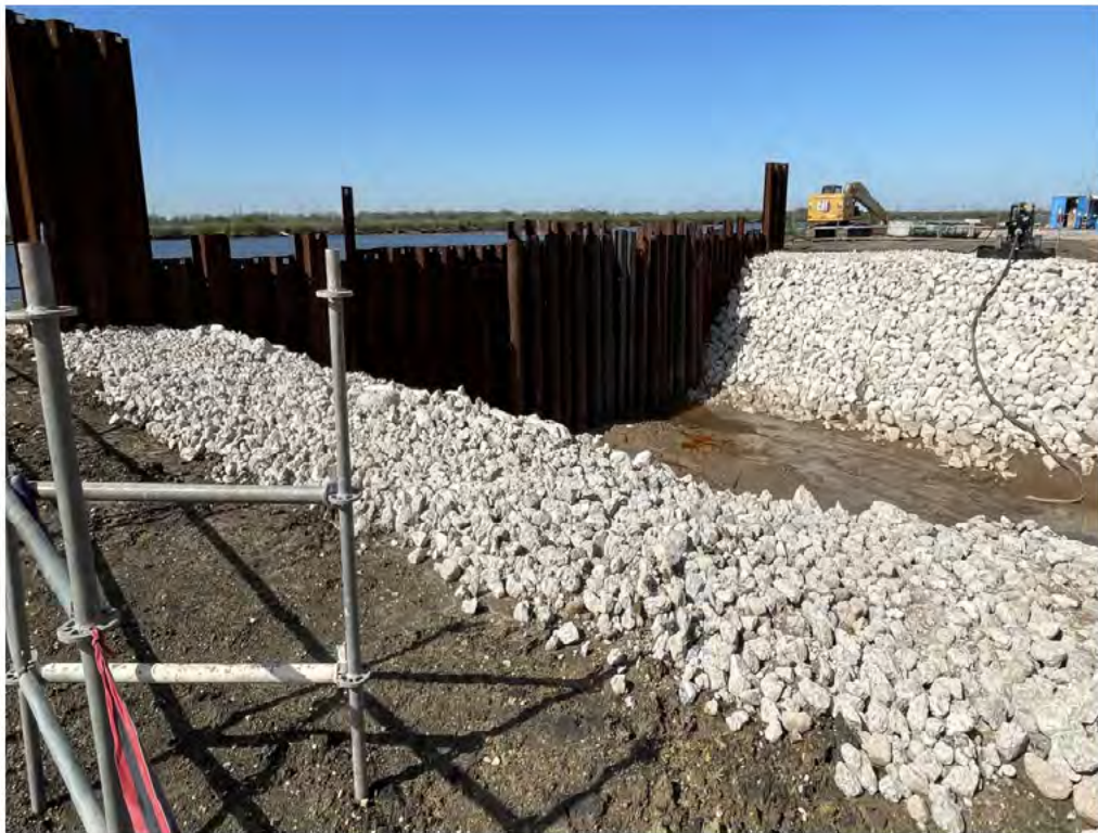
RWIS Repairs Completed – Channel & Rip Rap
