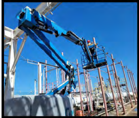
Nozzle Cleaning of Deluge System at BH PIG Trap Area
