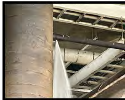
Leak at the Raw Water Intake Structure
